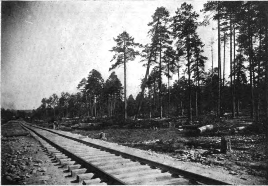
Tie Cutting Camp on the Orient.
